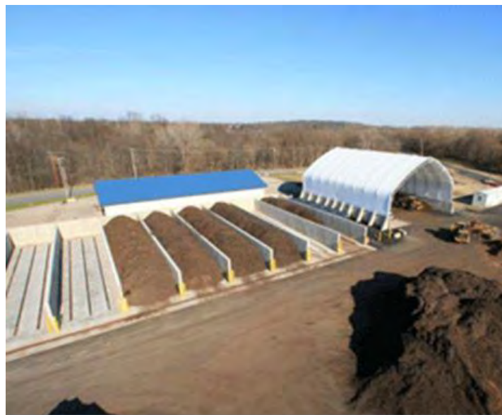
Onondaga County Resource Recovery Agency (OCRRA) Aerated Static Pile Operation
